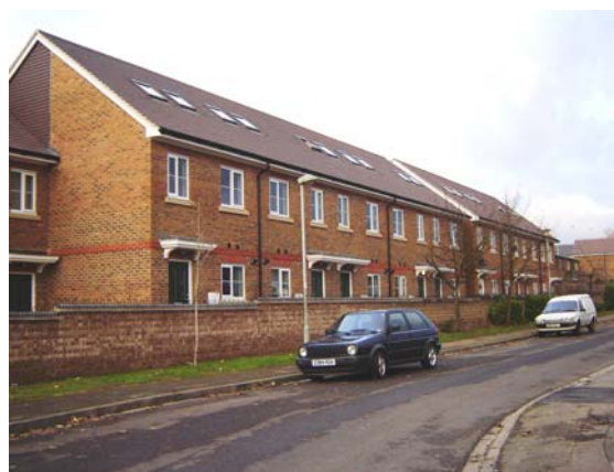
Affordable Housing at Saunders Road, Oxford
