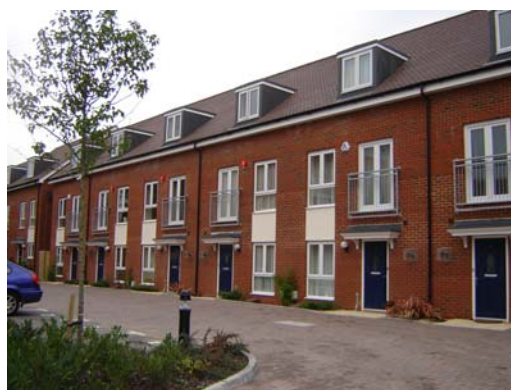
Affordable Housing at Rivermead Park, Oxford
